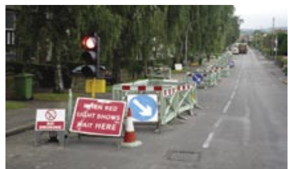
Utility highway excavations.
