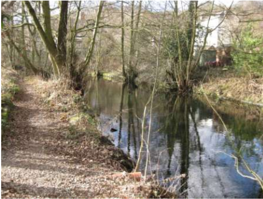
Section of canal in water between Sawmills and Bull Bridge
