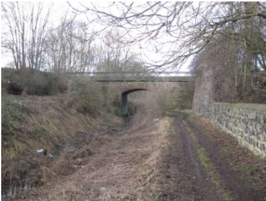
Lock No. 2 Bridge, showing retaining wall above towpath
