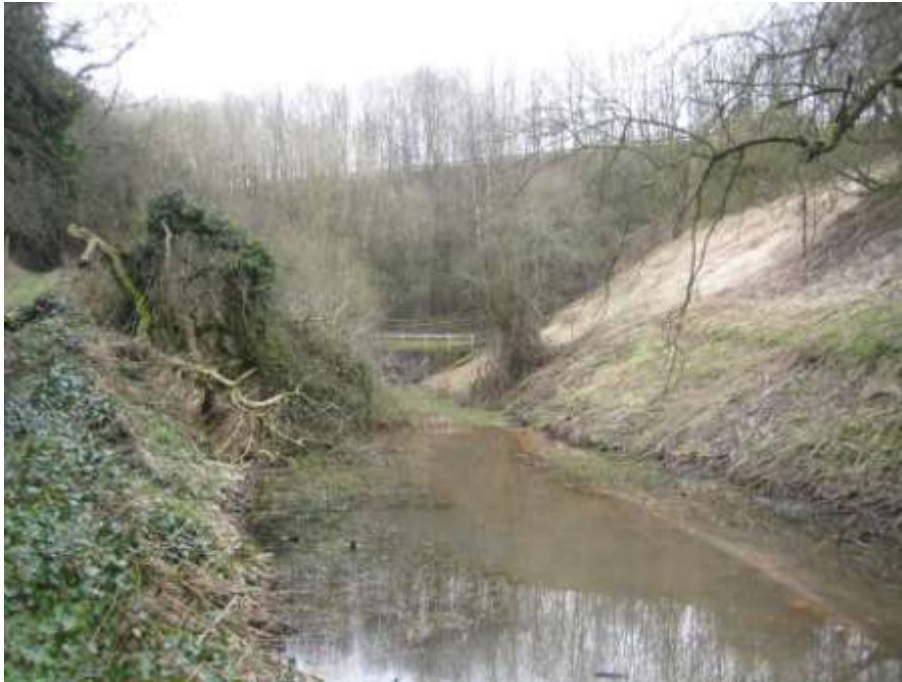
Canal between A38 and A610, looking back towards Butterley Tunnel West Portal and the A38 road
