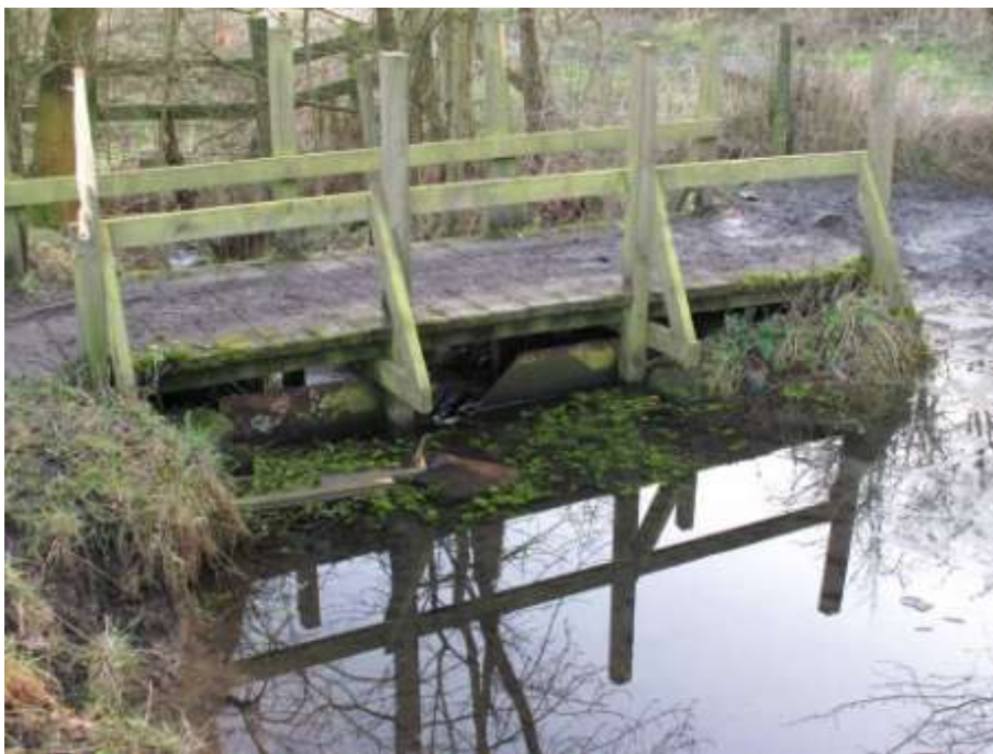
Footbridge with V-notch weir at site of LNER Bridge
