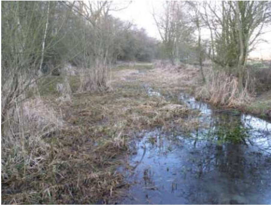
Course of Canal immediately north of LNER Bridge
