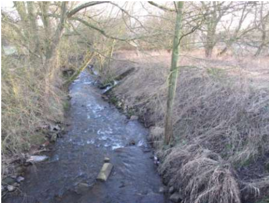
Weir (centre) discharging into River Erewash
