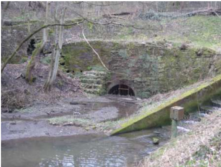
Tunnel East Portal and spillway
