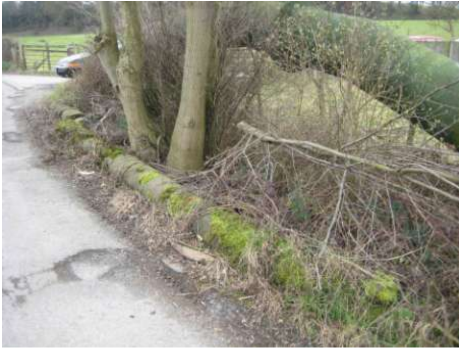
Pipe Bridge and parapet stones marking the site of Hartshay Bridge
