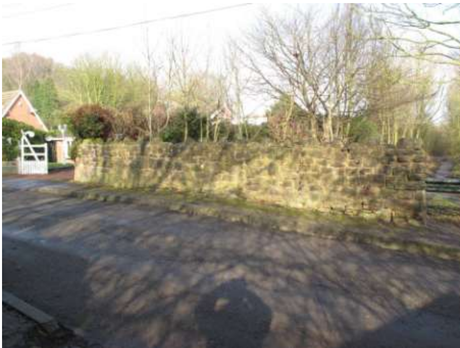
Site of Fletcher's Row Bridge, towpath continues towards Pinxton at approximately the same level as roadway
