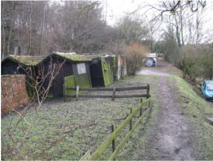
Encroachment onto the canal bed
