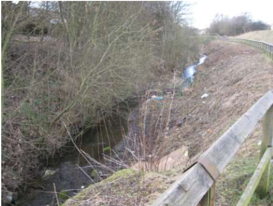
Final section of channel towards Pinxton Arm Junction and Codnor Park Reservoir, in deep cutting to provide flood route for Codnor Park Reservoir
