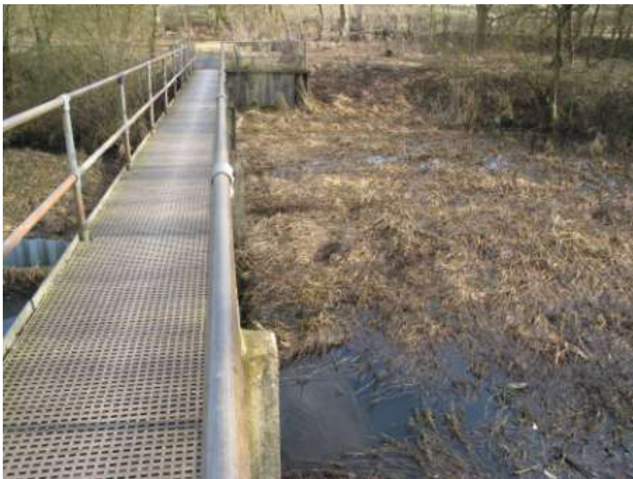
Reservoir inlet weir and footbridge
