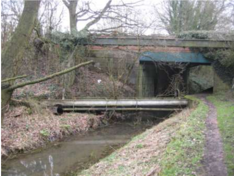
Ripley Road Bridge
