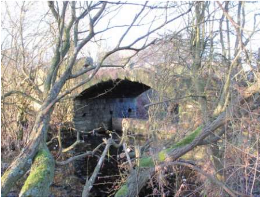
Portland Basin Bridge – the arm to the basin passed under the bridge
