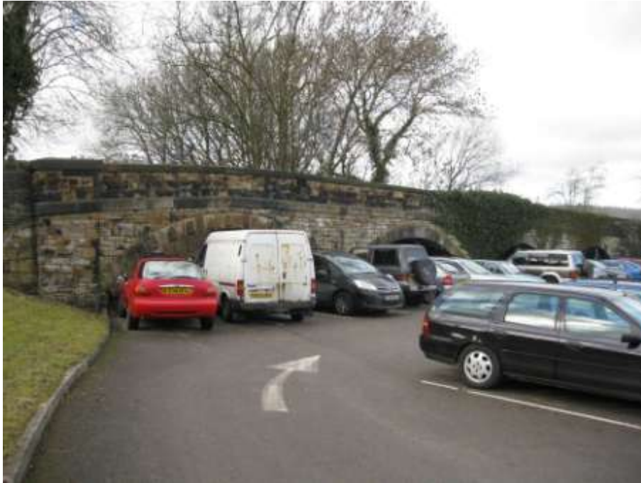
Brick Yard Bridge
