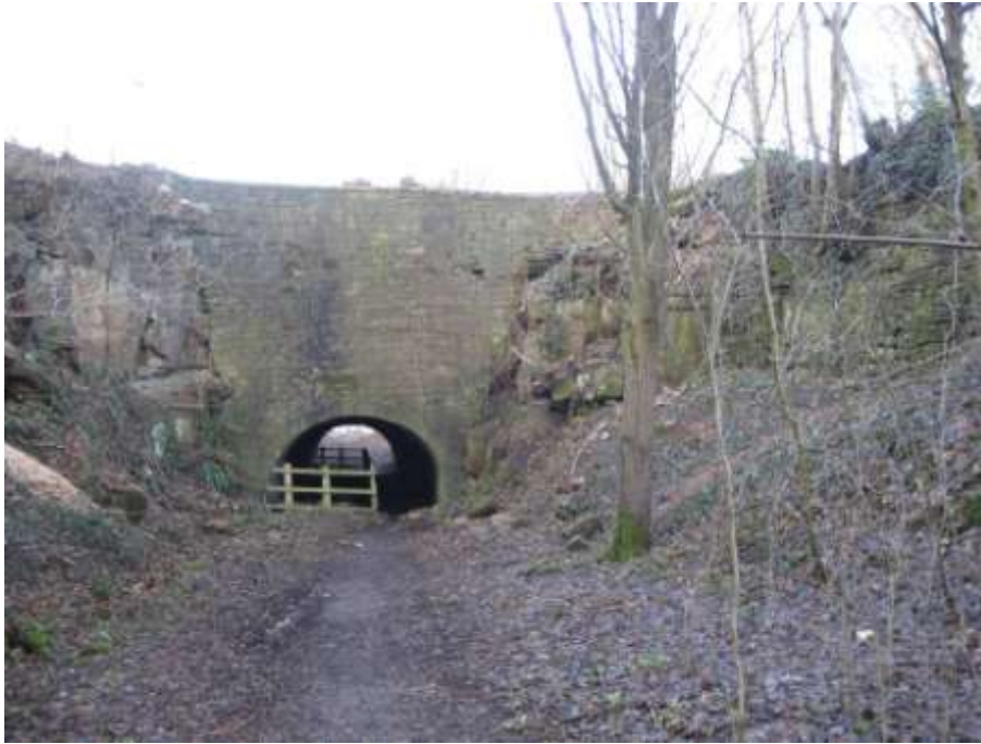
Buckland Hollow Tunnel
