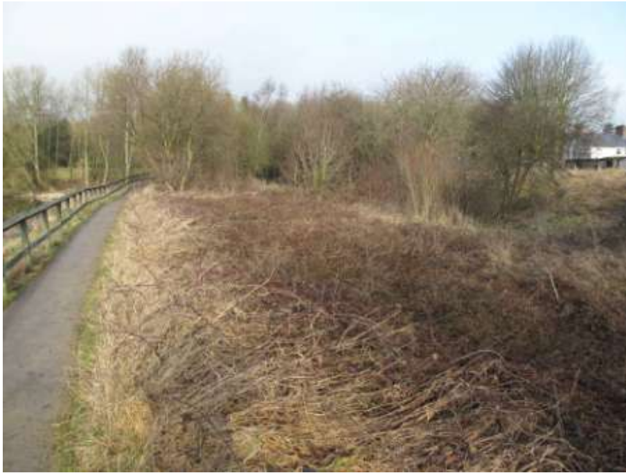
Channel across Codnor Park Reservoir dam
