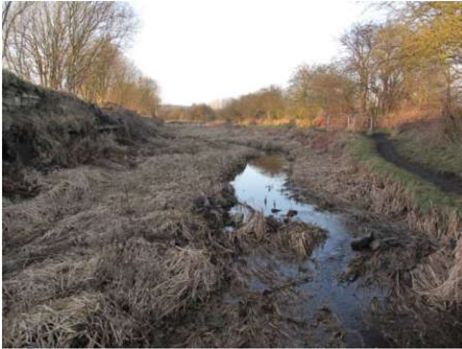
Canal north of Portland Basin Bridge, with remains of Butterley Company wharf buildings on left
