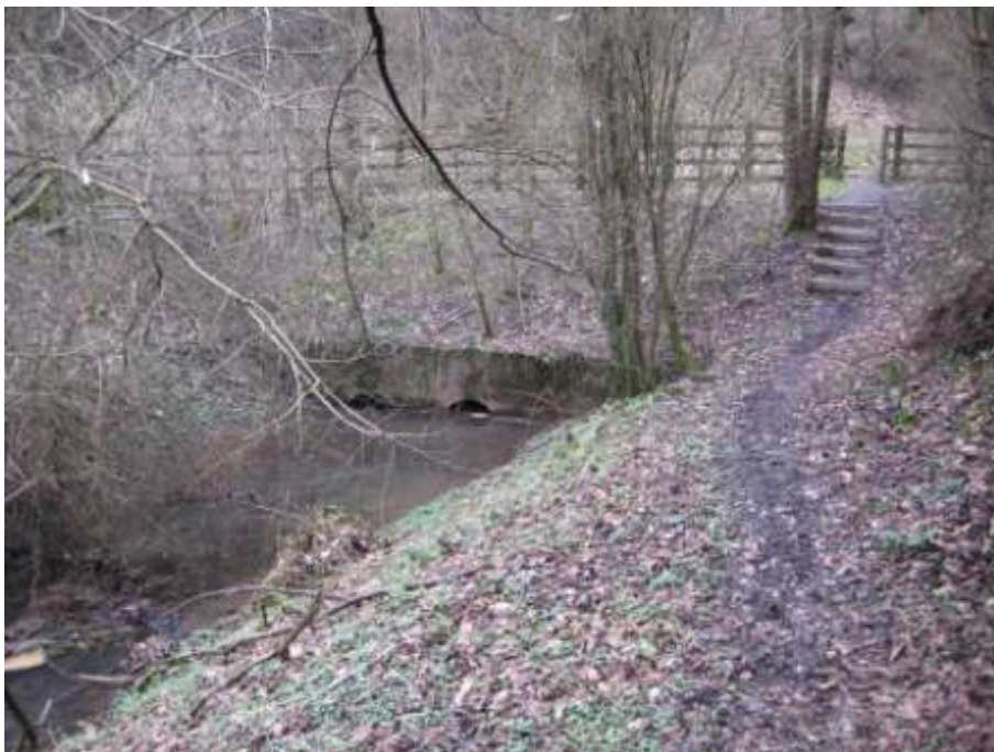
East end of culvert under A610
