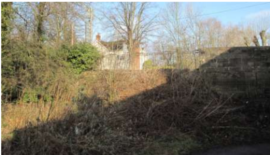
Pye Bridge (infilled, but apparent from railings)
