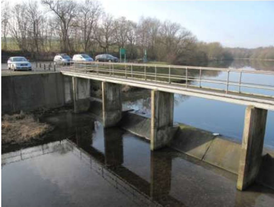
Codnor Park Reservoir Outlet Weir – canal was located where car park is
