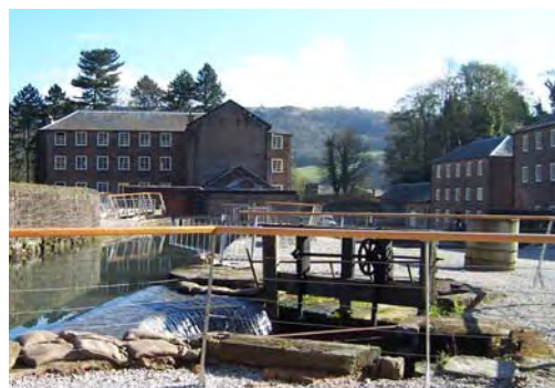
The Canal starts here in the yard of Arkwright's Cromford Mill where a sluice diverts water into a culvert under the buildings and via a feeder arm to the Wharf across the road.
