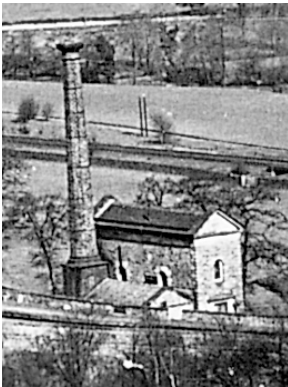
Leawood Pumphouse pre-1916
