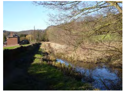
A narrow channel through vegetation must be kept open at the Ambergate end so that water and silt can get away
