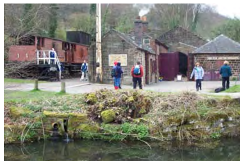
The very early example of railway workshops at High Peak Junction and the bottom of the first inclined plane of the Cromford and High Peak Railway.
