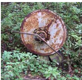
Signalling equipment at the bottom of Sheep Pasture incline which communicated to the winding engineman at the top of the incline.
