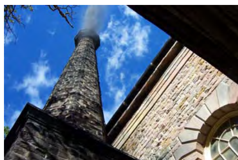
One gain from the railway takeover was the building of the magnificent Leawood Pumphouse to pump water from the Derwent up into the Canal. Volunteers continue to steam up the Leawood Pump on regular open days.
