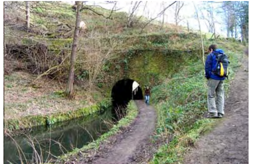
Gregory Tunnel from the north. Fully-lined and 40 yards long, despite the hilly terrain, this is the only tunnel along the Derwent Valley length.
