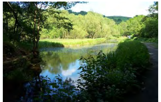
Gregory Winding Hole from the tunnel mouth with the cliffs and monument of Crich Stand on the horizon. The canal retaining wall here is doing the job of a dam, collecting water from the streams which drain the hillside above. The richest habitat for aquatic communities on the Canal is here, but dense vegetation is fast encroaching on the area of open water and degrading the habitat.
