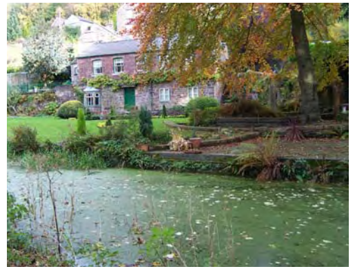
The sawmill building at Robin Hood, with the rim of the stone-lined pit visible to the right. The gardens cover the extensive wharf area.
