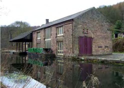
The Wharf Shed (transhipment warehouse) at High Peak Junction.
