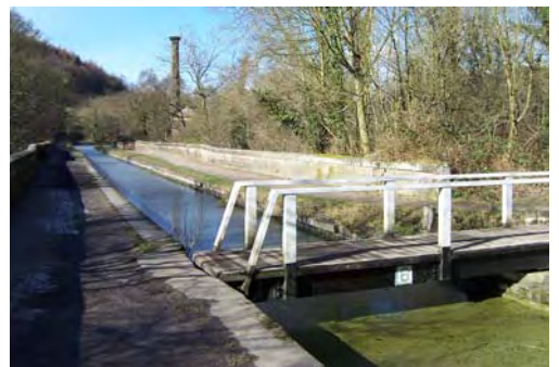
The Canal narrows at the Derwent Aqueduct and the towpath changes side over a swing bridge. The chimney of the Leawood
