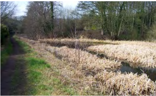
Calladine Winding Hole, between Poysers and Grattons Bridges, where boats could turn. Potentially a good aquatic habitat, it has been degraded, like the rest of the Canal, by vegetation encroachment, low water levels and lack of a through flow.
