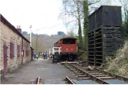
High Peak Junction Workshops, demonstration track and wagon. The water tank (right) supplied domestic fresh water to villages up the line and served the engines.
