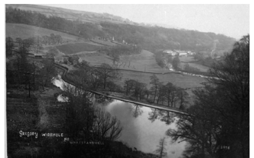
Gregory Winding Hole in times past, with the remains of the old boat docks visible beyond the basin. These are now overgrown as is a large proportion of the open water area visible here. The dam construction was also much more legible before vegetation took hold on the downhill side. Restoration work will benefit wildlife and the constructed environment equally.
