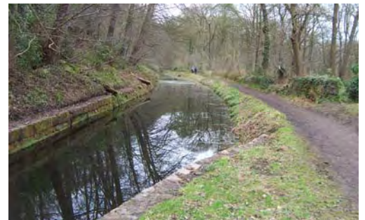
Generally stone edges to the Canal are found at wharfs and either side of bridges. Here, the Canal narrows for a wharf or crossing place some distance from any obvious activity or route.
