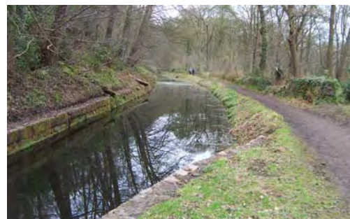
Generally stone edges to the Canal are found at wharfs and either side of bridges. Here, the Canal narrows for a wharf or crossing place some distance from any obvious activity or route.
