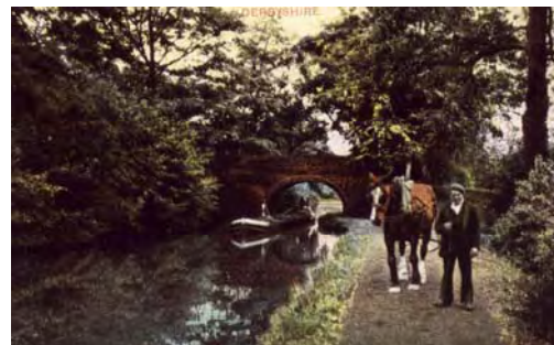
This postcard of a horse-drawn canal boat passing under Chase Bridge illustrates the width the towpath will have been along the length of the canal— wide enough for two horses to pass.
