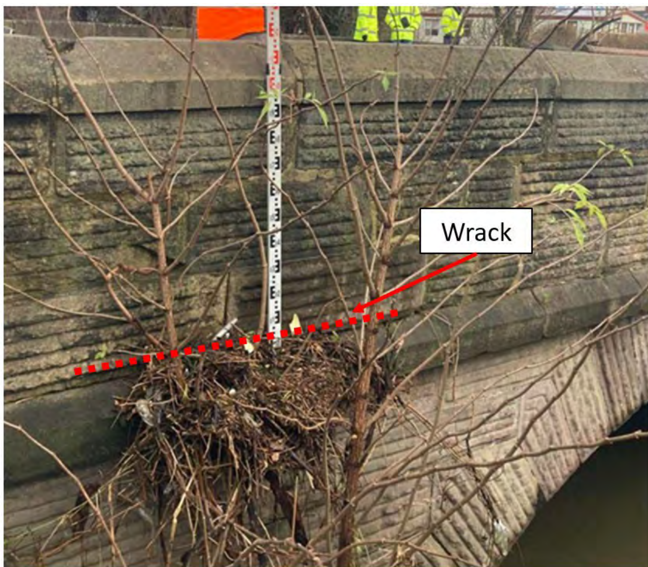
Figure 7-22: Wrack mark on the upstream face of Derby Road bridge. Source from the Environment Agency.
