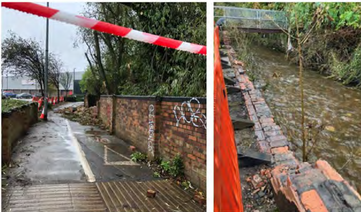
Figure 4-24: Collapsed walls as a result of the overtopping of Holme Brook (left) and the Hipper (right).
