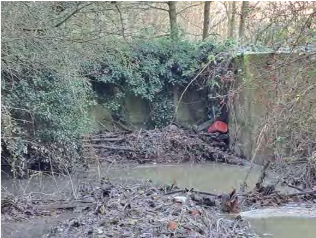
Figure 4-33: Debris blockage at Smithy Brook culvert inlet (upstream of Smithy Brook Road).
