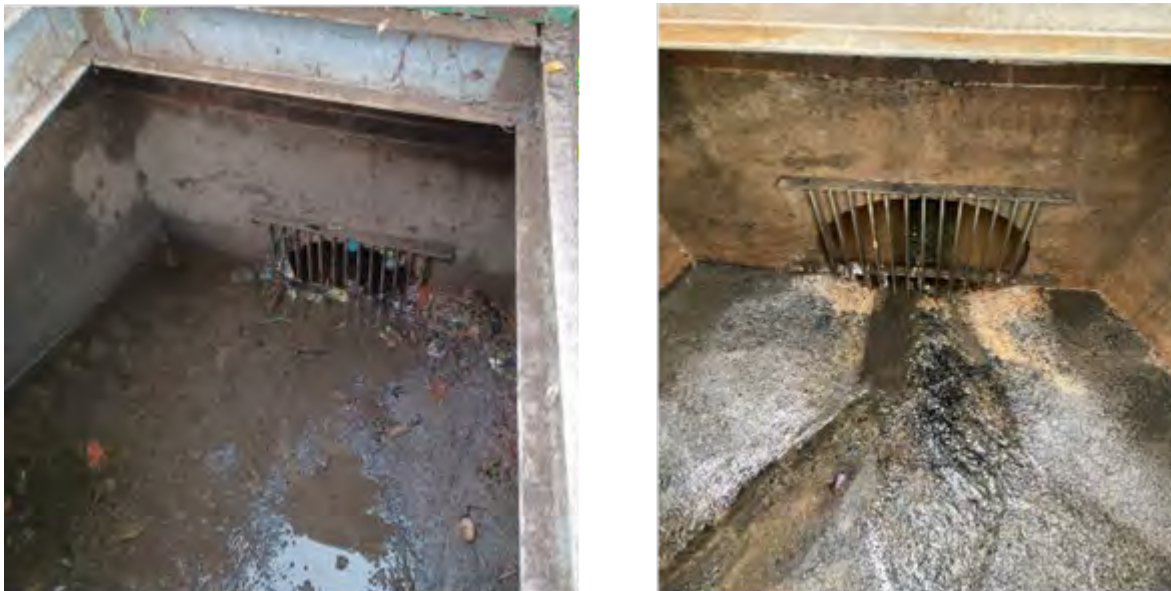
Figure 3-5: The picture on the left shows the chamber before cleaning and after de-silting on the right.
