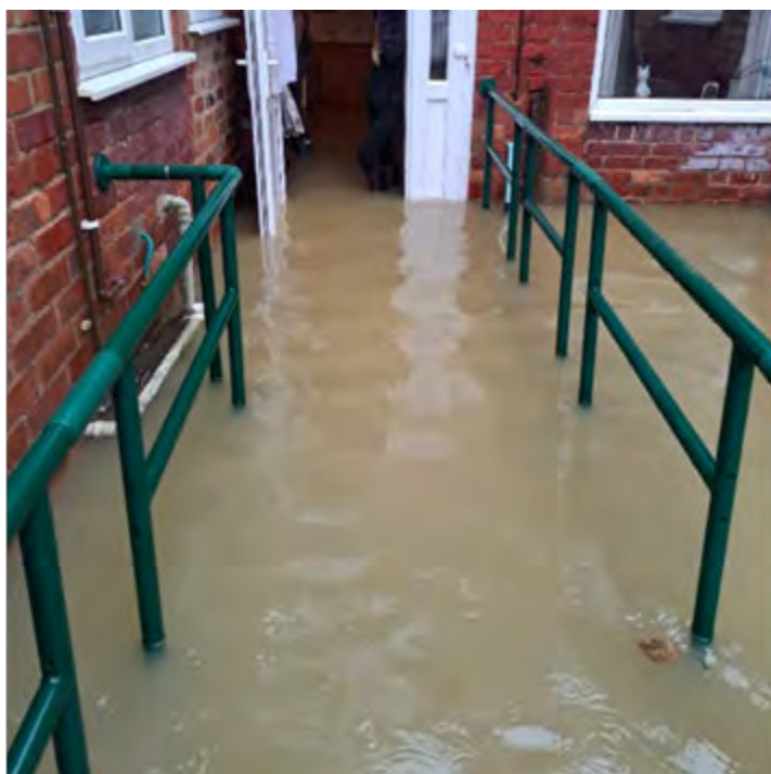
Figure 7-29: Flooding to a property in York Terrace.
