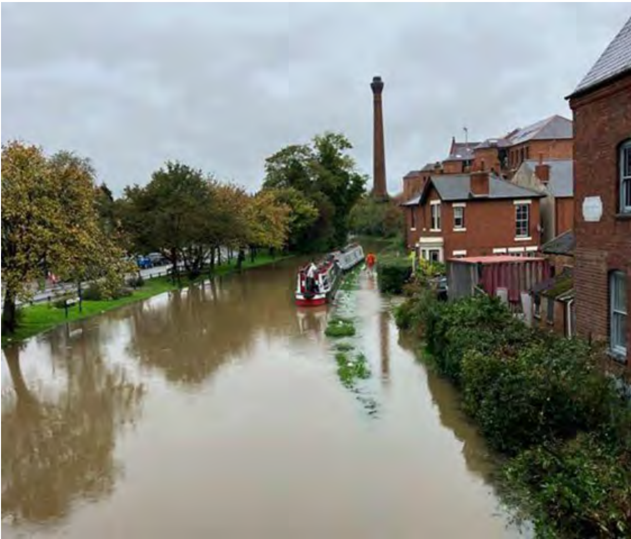
Figure 7-13: Flooding of the Erewash Canal: The River Erewash overtopped, and fluvial flood water entered the Erewash Canal which acted as a conduit for the flood flow.
