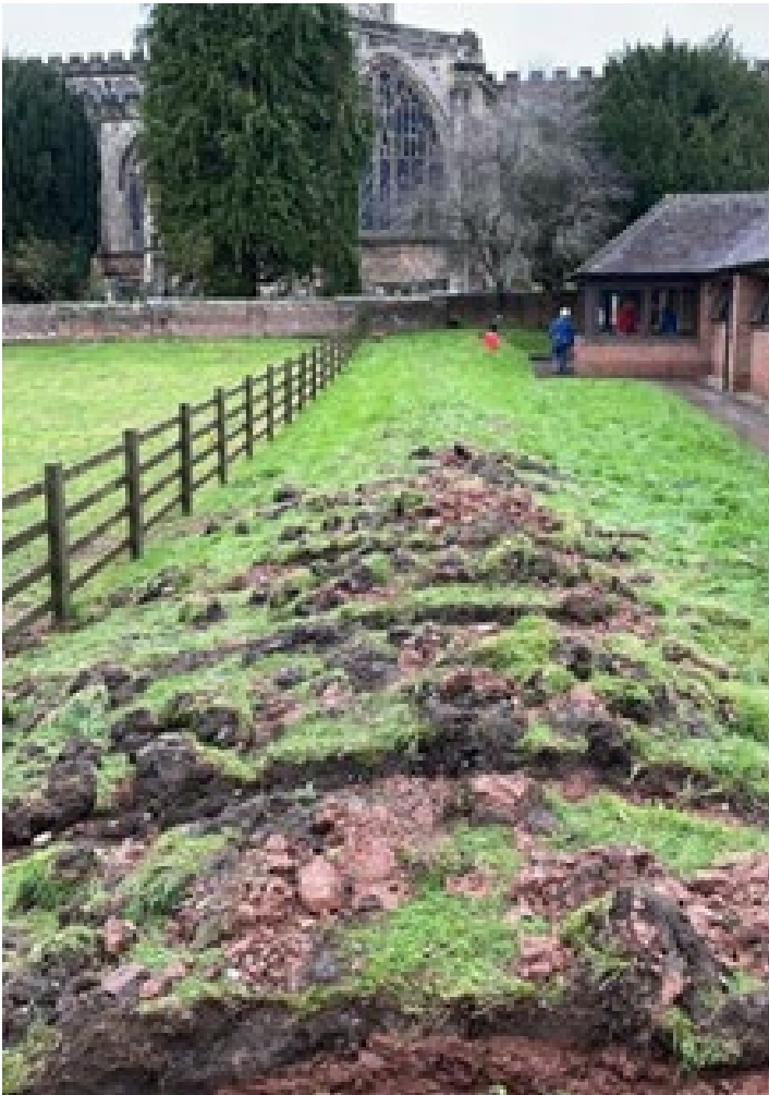
Figure 5-6: Channels were excavated into the flood embankment to the west of St Oswald's Church Hall to allow water to escape.
