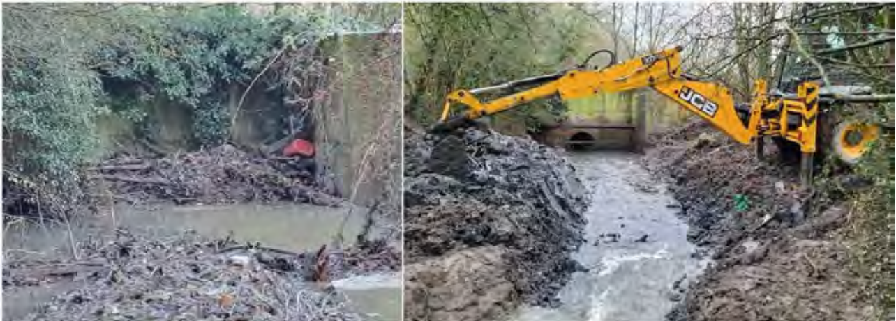
Figure 4-34: Smithy Brook culvert prior (left) and post (right) trash screen clearance.
