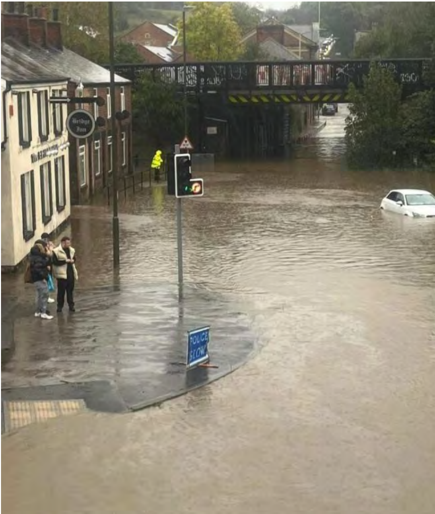
Figure 4-46: Flooding on Hollis Lane, facing eastwards towards Hady Hill.
