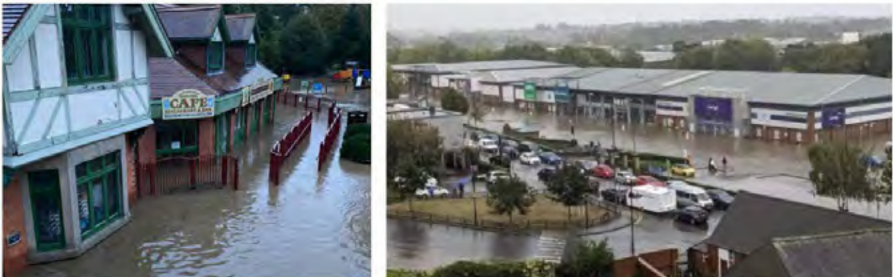
Figure 4-43: Left - Flooding at a business within Queens Park. Right - Flooding on the northern side of Ravenside Retail Park.
