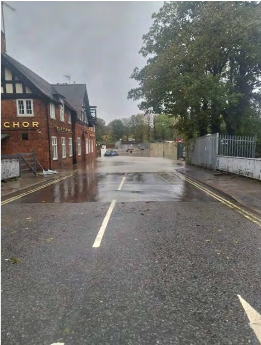
Figure 4-23: Flooding of low spot on Factory Street. Photograph taken from immediately north of Factory Street bridge.
