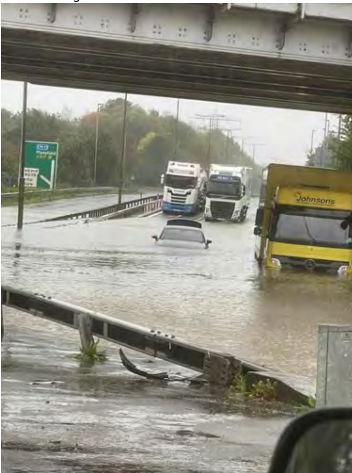
Figure 4-44: Flooding on the A617 at the low spot beneath the railway underpass at Horns Bridge. Photograph taken from Horns Bridge Roundabout.
