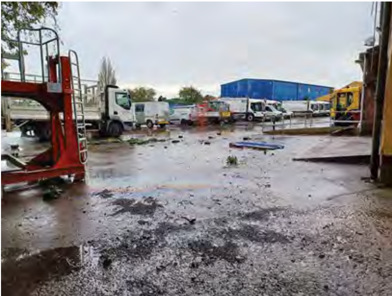
Figure 4-55: Eckington Depot affected by flooding because of Storm Babet.
