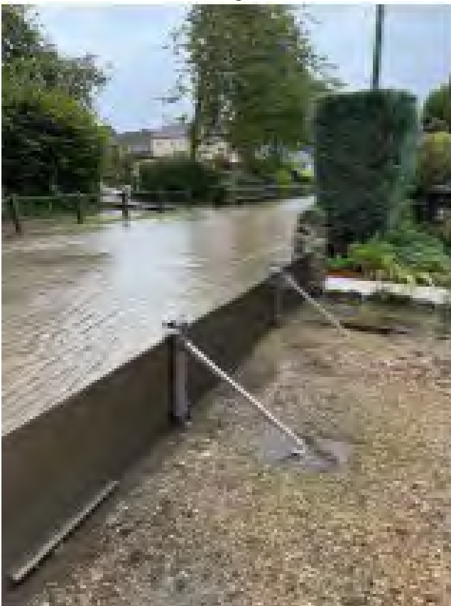
Figure 3-28: Demountable flood barrier across a driveway prevents flood water reaching a property in Breadsall.
