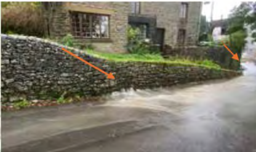
Figure 3-46: Surface water runoff flowing through a drystone wall and onto Brookside.
