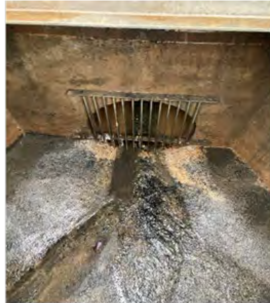
Figure 3-5: The picture on the left shows the chamber before cleaning and after de-silting on the right.
