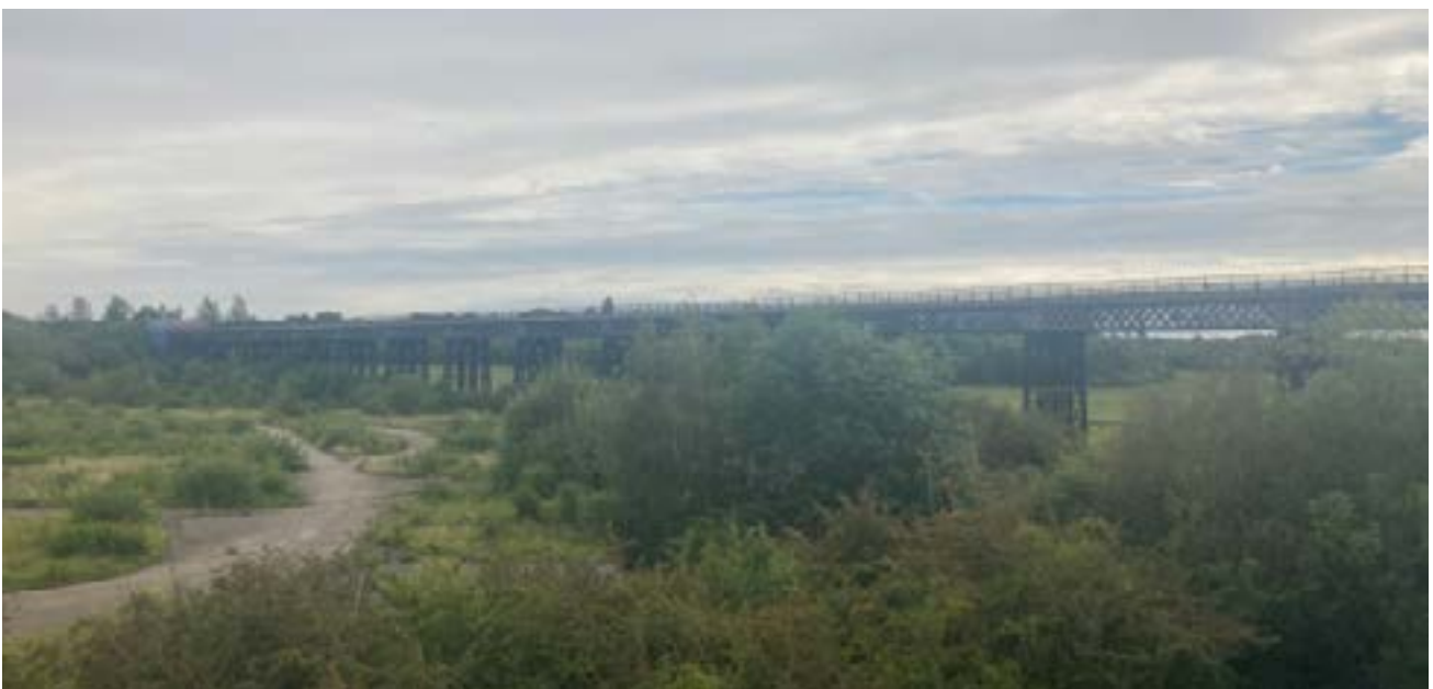
Figure 32: The Bennerley Viaduct, as seen from the viewing platform
