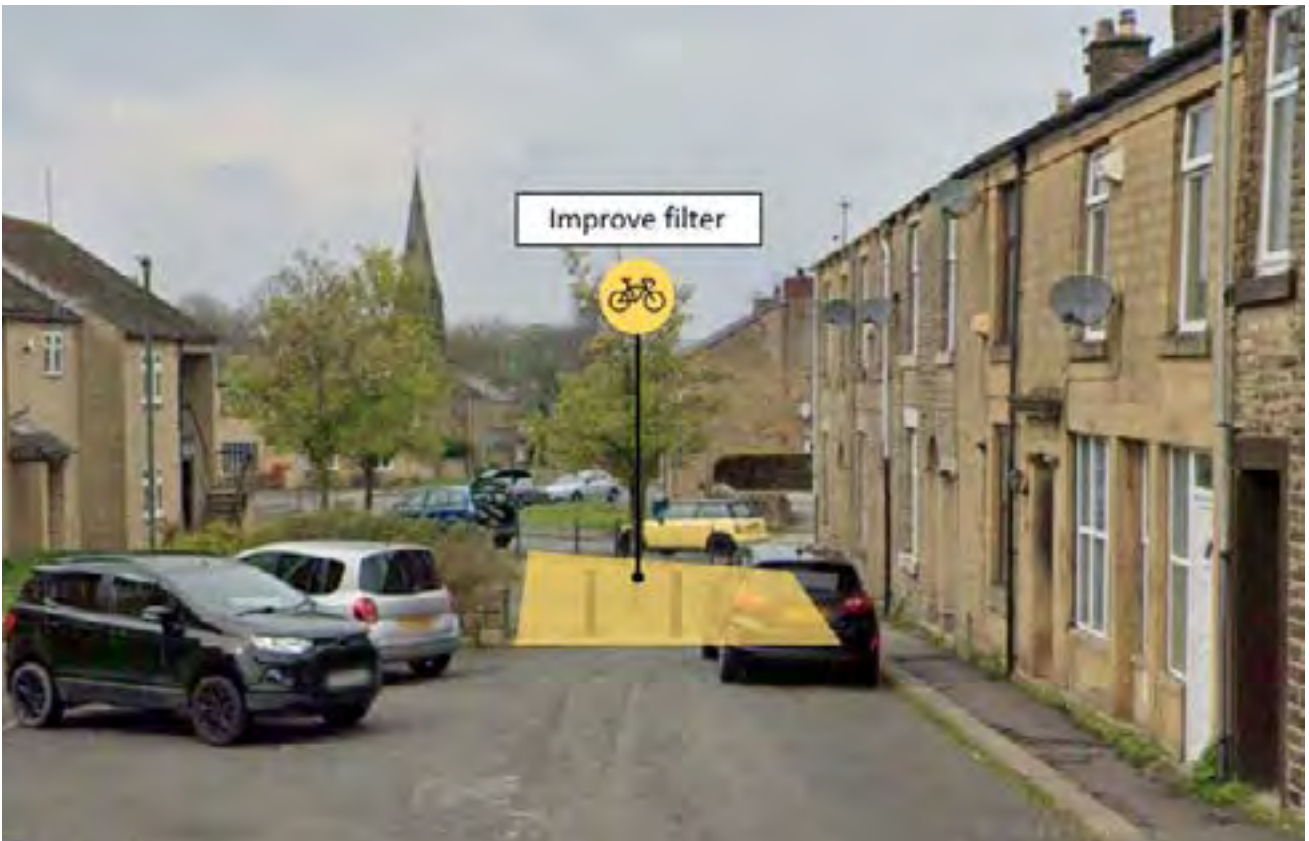
Figure 27: Example of an existing road closure on Freetown
