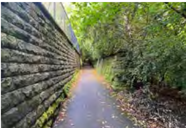
Figure 16: Existing ramped path within Manor Park
