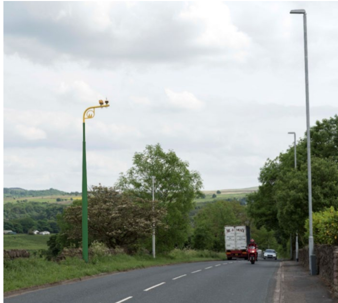
Photograph showing an alternative green colour column with yellow camera support arm, which has been used in a number of areas of Outstanding Natural Beauty. This colour has received some criticism for being camouflaged, as the column can seem to disappear if surrounded by foliage.
