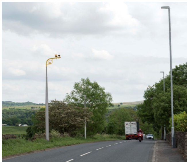
Photograph showing an alternative grey column colour with yellow camera support arm which has been used in a number of National Parks (The Trossachs, Cairngorm) and in Cumbria. Overall, the conspicuity is reduced, but there is still a visible presence.
