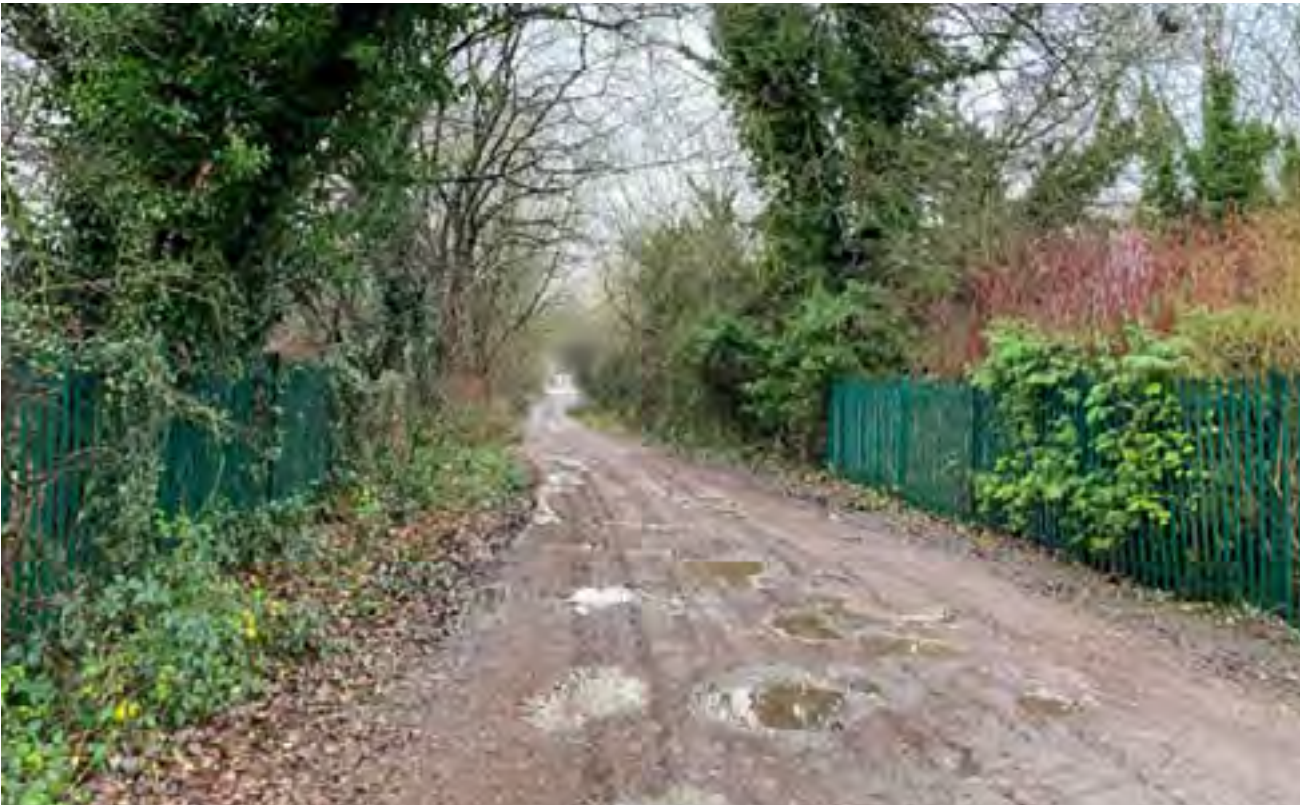
Figure 34: Existing surface between Simmondley Lane and Adderley Road
