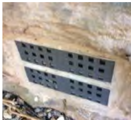
Self-closing airbricks.
