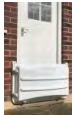
Electric sockets further up the walls, barriers to all external doors and non-return valves fitted.
