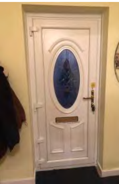
Flood resilient front door has been installed.
