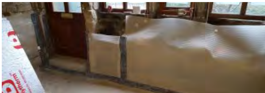
Waterproof membrane during installation.
