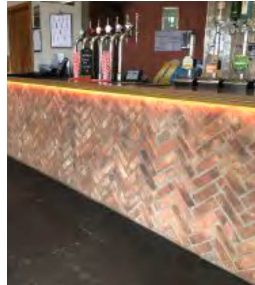
The bar is now brick and has been treated with a waterproof spay. The floor is tiled.
