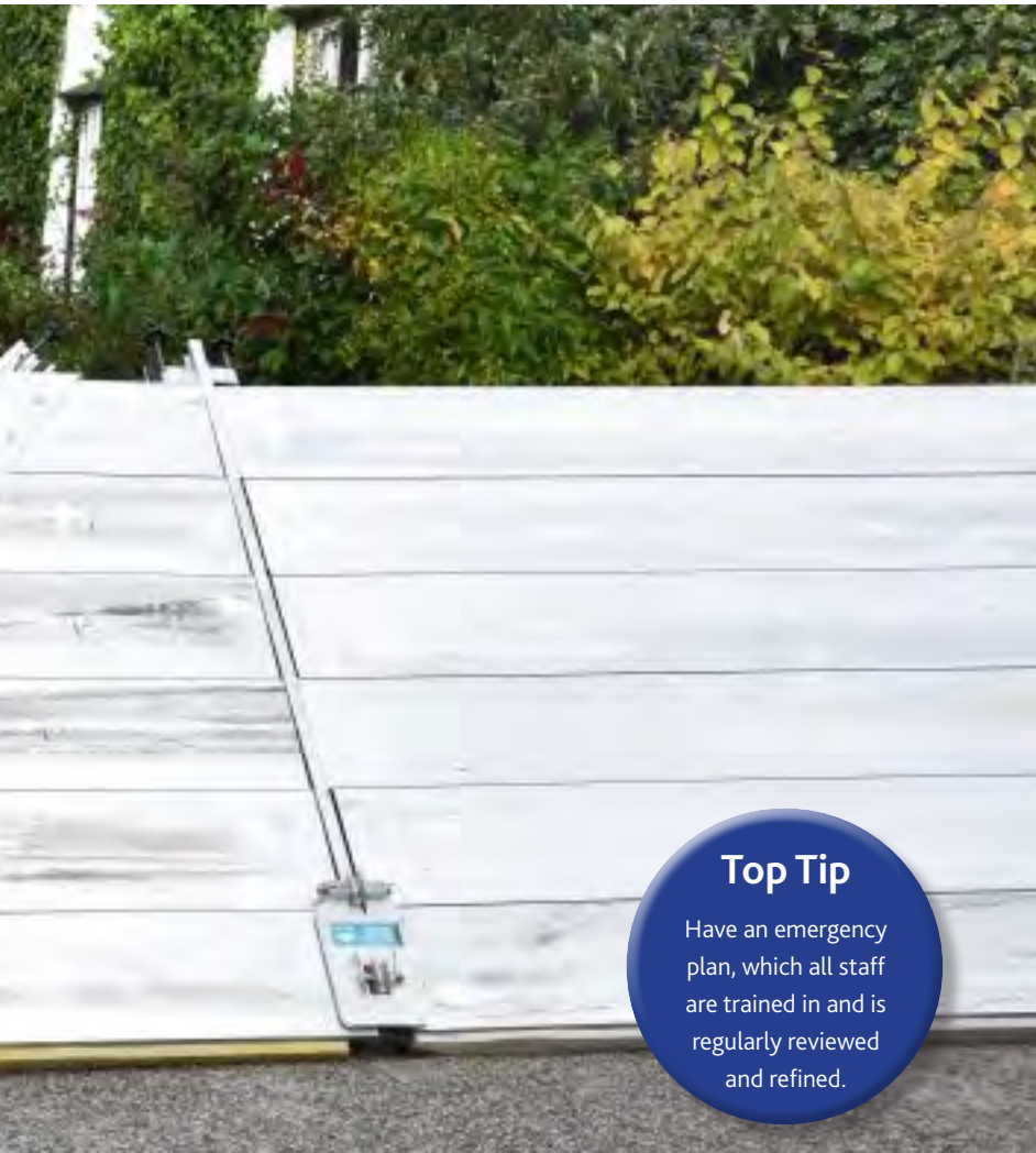
Rigid temporary barriers are installed around the hotel to a height of 1.2 metres. The hotel has 'Flood Marshals' trained to put the barriers in place, which take 6 people about 1.5 hours.
