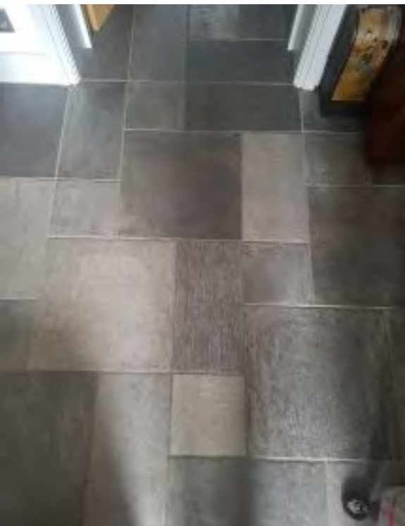
Tiling in the ground floor above insulation and underfloor heating.
