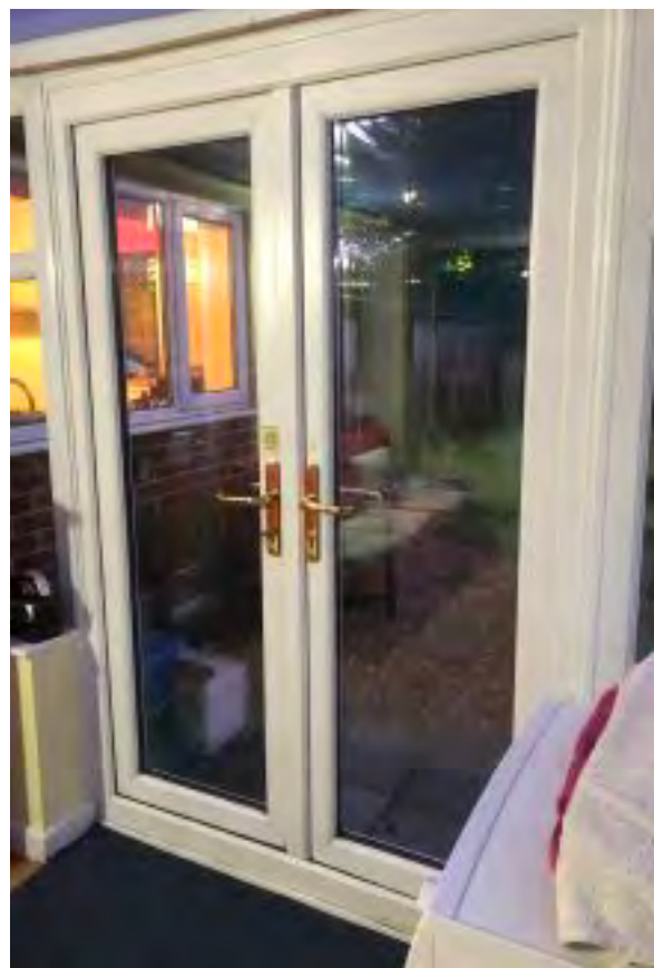
Flood resilient patio doors have been installed.
