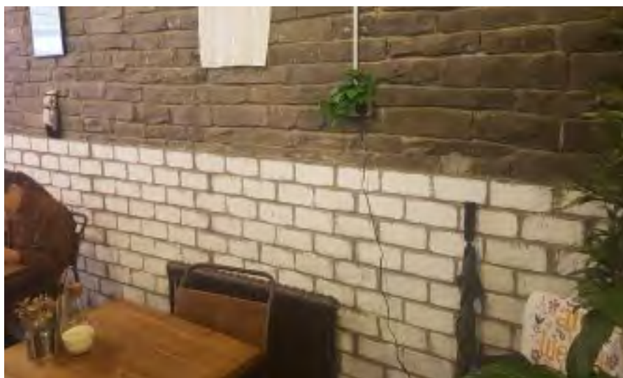
Walls stencilled and painted to resemble tiling.
