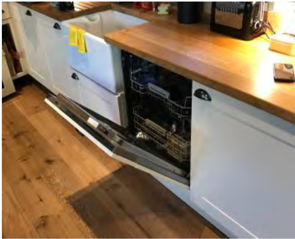
Existing kitchen and floor finishes were removed, and then re-installed following completion of the work.
