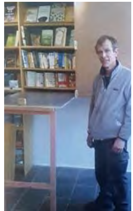
Wall shelves fold up, and legs are inserted to create tables for storing stock from lower levels.
