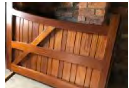
Solid wood gates to be fitted onto metal posts.
