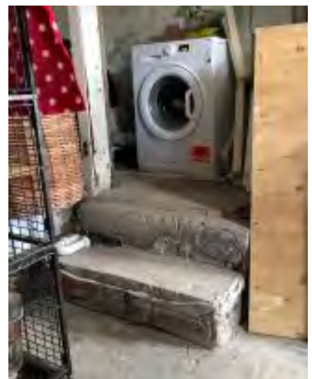
White goods in the basement room are now raised up.
