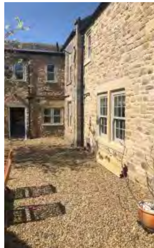
Permeable patio areas surround most of the house.
