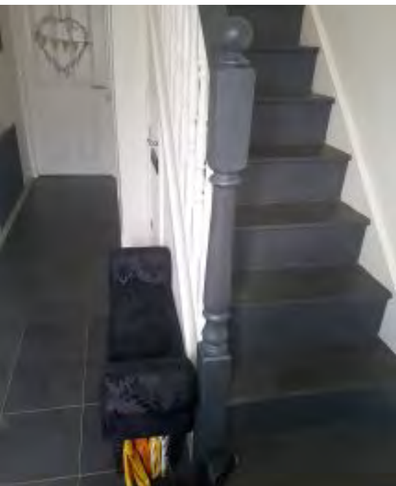
Tiling in the hall floor using waterproof adhesive and grout and removed stair carpet.
