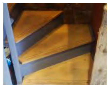
Steel staircase and solid oak treads.
