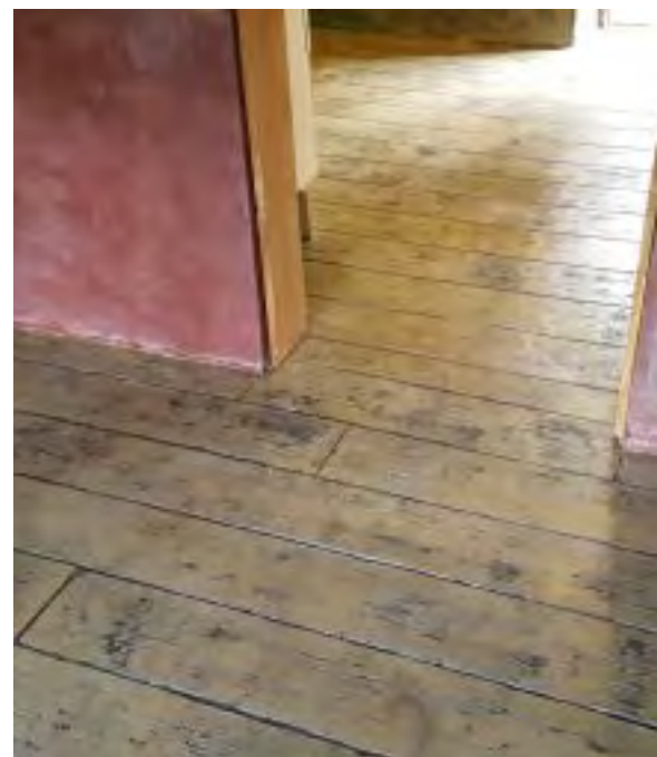
The floor is concrete, with an antique wood effect pattern, and sealed to give a gloss finish.
