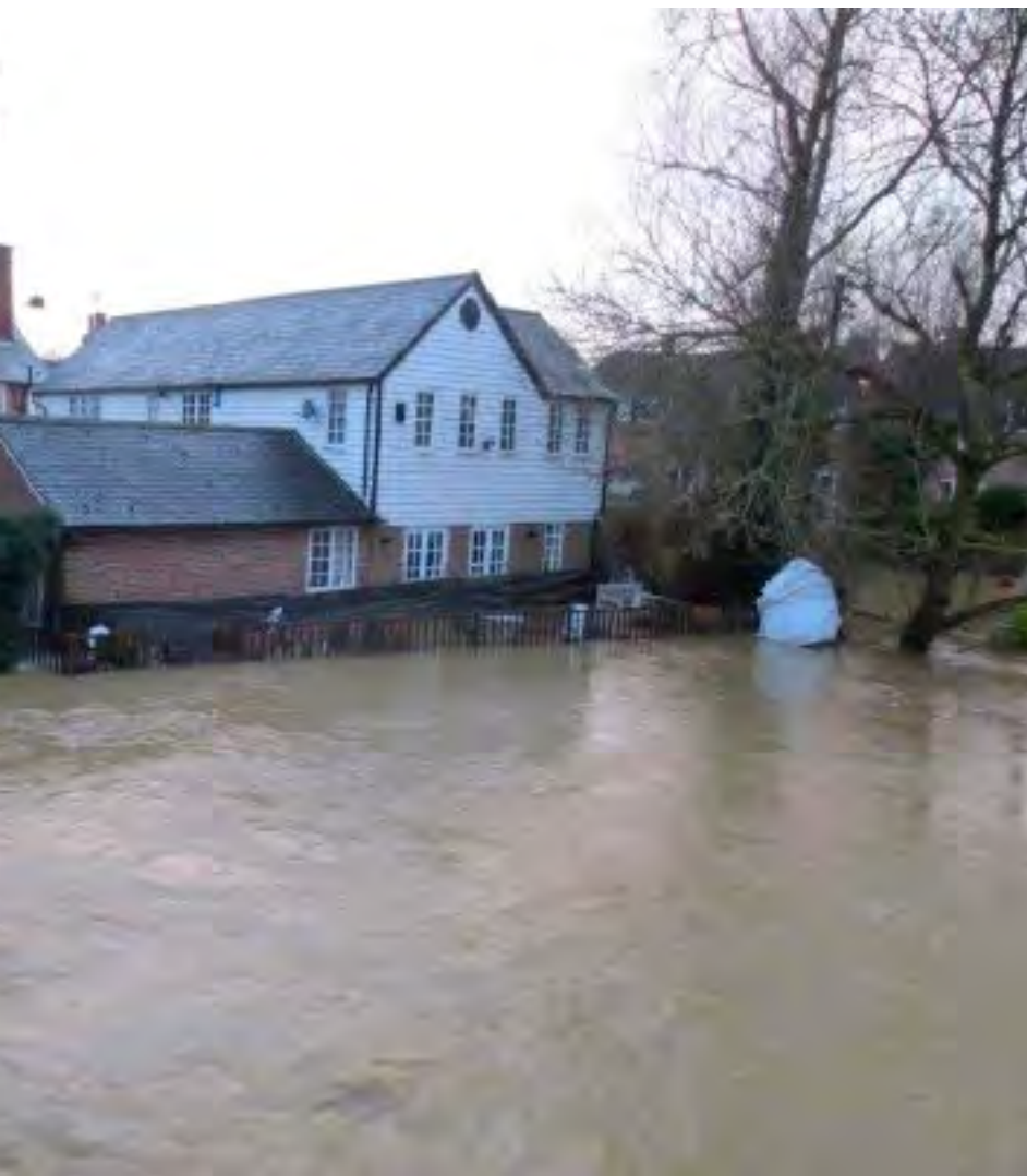
The building skirt system usually coped quite admirably and no water entered the property until it was overtopped in 2013.
