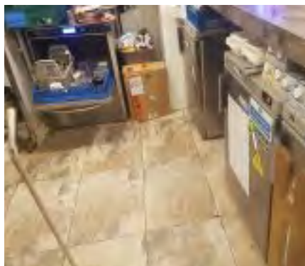
Tiled kitchen floor with waterproof adhesive and grout.
