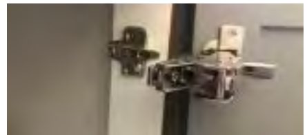
Kitchen doors have easy release hinges, so the doors can be removed quickly.
