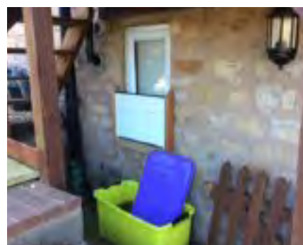
Flood barrier to basement door and window.
