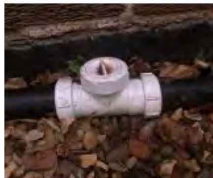
Non-return valve in pipework, to prevent backflow.
