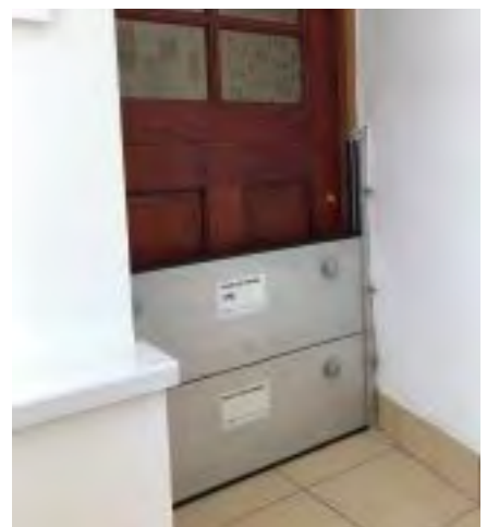
Flood barriers to all external doors and tiled floors.
