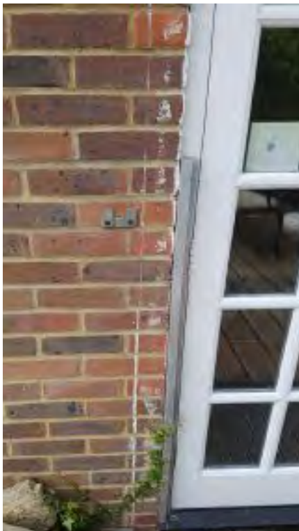
External hook on the wall that holds the building skirt system.
