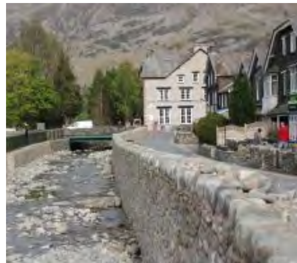
Newly upgraded Environment Agency defences.
