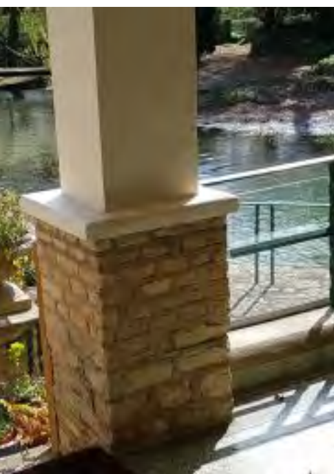
The glass barrier with floodgate for access on river-facing side.
