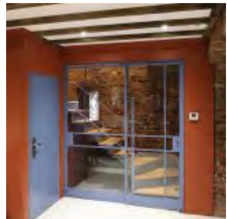
Glazed sliding door/screen in powder-coated steel.
