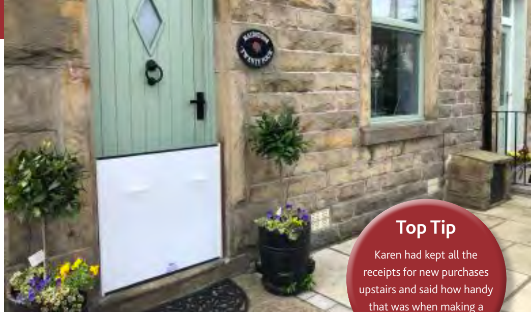
Flood Barrier to basement door and window.
