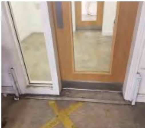
Flood barriers to all doors and UPVC door architraves.
