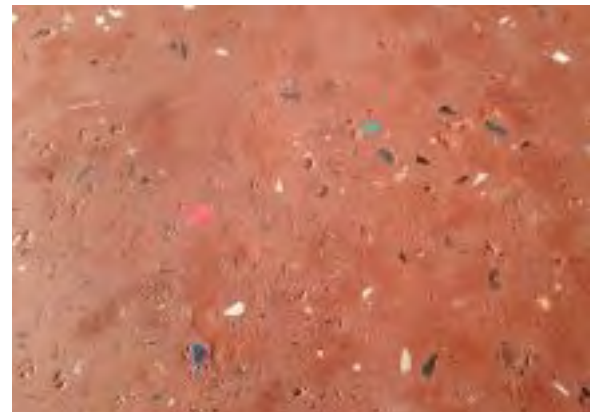
The walls were rendered using coloured renders.
