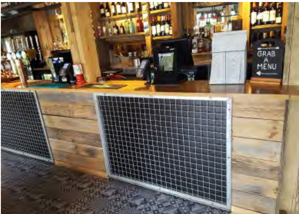
The fixtures are made of old reclaimed wood, which can be washed and salvaged.
