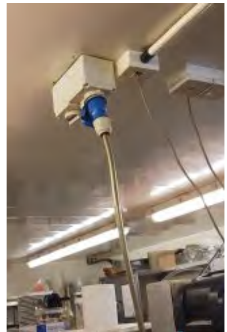
The electricity and gas supply are high up and can be easily turned off and back on.
