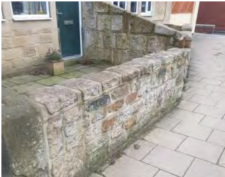
New wall at front of house with a flood-proof gate
