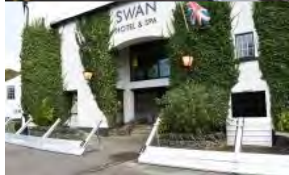
Rigid temporary barriers are installed around the hotel to a height of 1.2 metres. The hotel has 'Flood Marshals' trained to put the barriers in place, which take 6 people about 1.5 hours.
