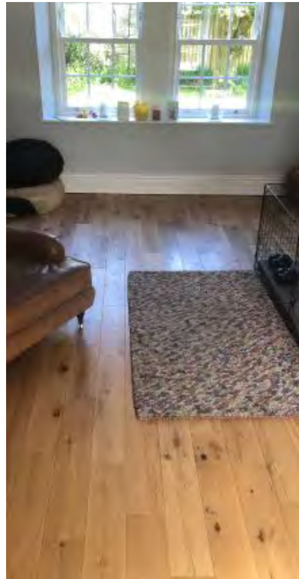
Engineered oak to the remaining floors.
