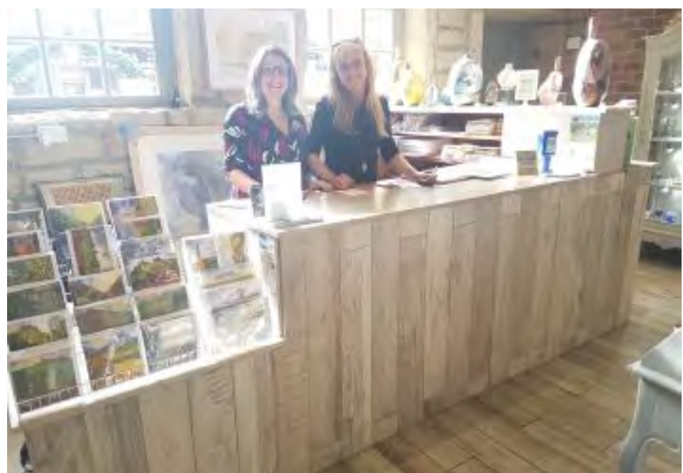
Counter base and new shelving is made from marine ply and coated with sealant.
